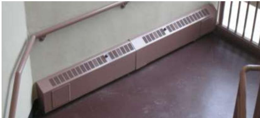
**Figure 2.6: Wallfin Convectors in Stairwells**
