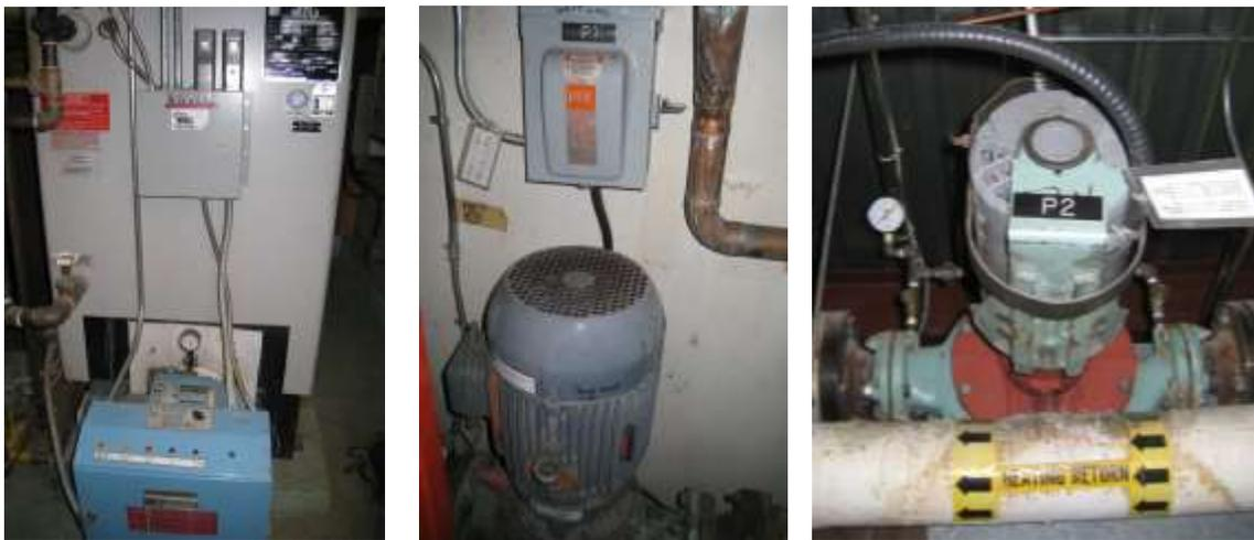
**Figure 2.5: Existing BRYAN Natural Gas Boiler & Circulation Pumps P1 & P2**
