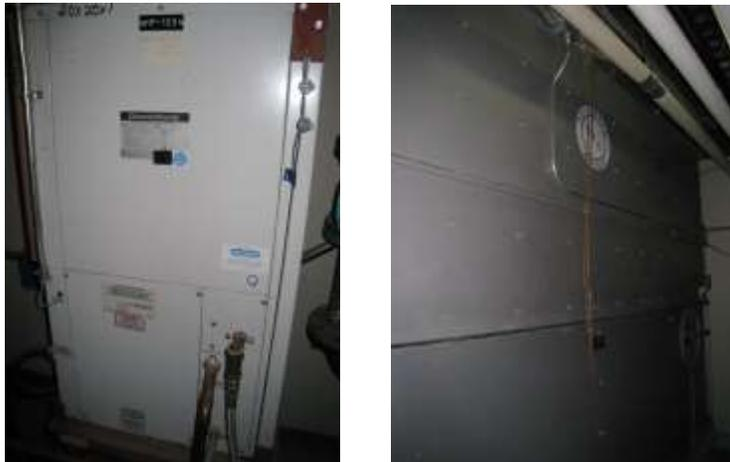
**Figure 2.7: Heat Pump and Fluid Cooler**
