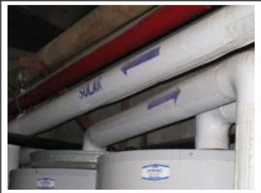
A photograph showing a mechanical room with several large white cylindrical tanks. White pipes are connected to the tanks, with the word 'SOLAR' and blue arrows hand-painted on them to indicate flow direction. A red-painted pipe is visible at the top of the frame. |
