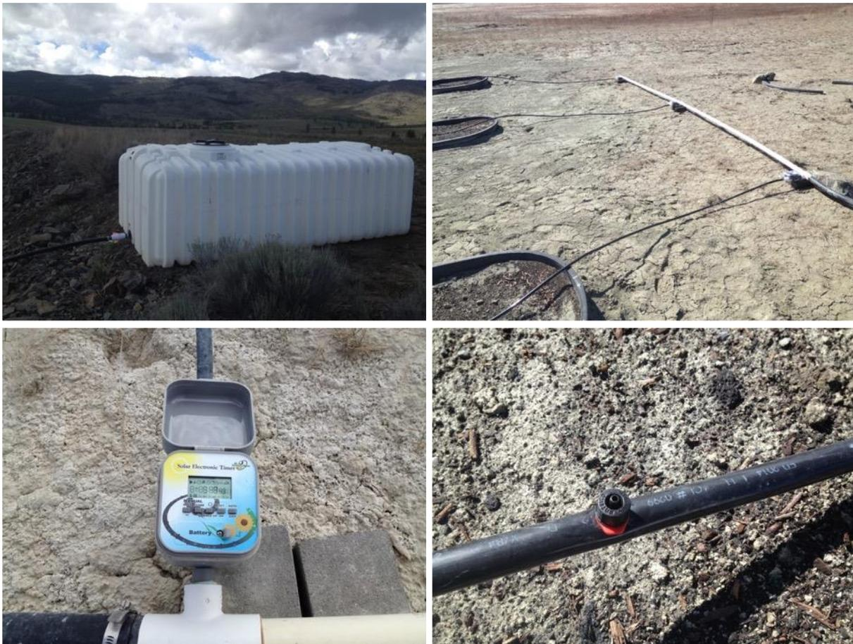
**Figure 3.6.** View of automatic gravity feed drip irrigation system installed at the Historic Afton Tailings Storage Facility research site in 2015. A 2000-gallon water tank elevated on the tailings dam (top left), 3-way independent water delivery system (top right), low pressure automatic irrigation timer (bottom left) and ½ gallon/hr. drip nozzle (bottom right).
