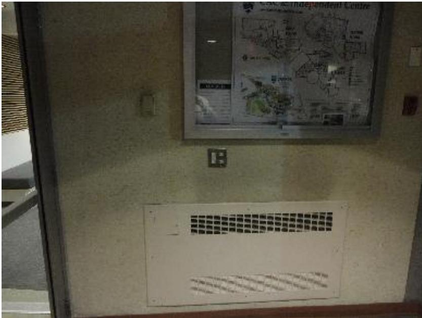
Figure 3: Forced Flow Heater in Vestibule
